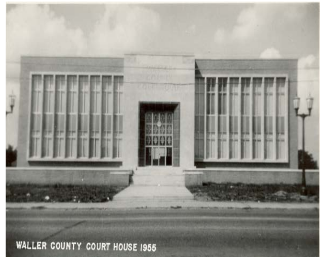
Figure B.2: Waller County Courthouse
